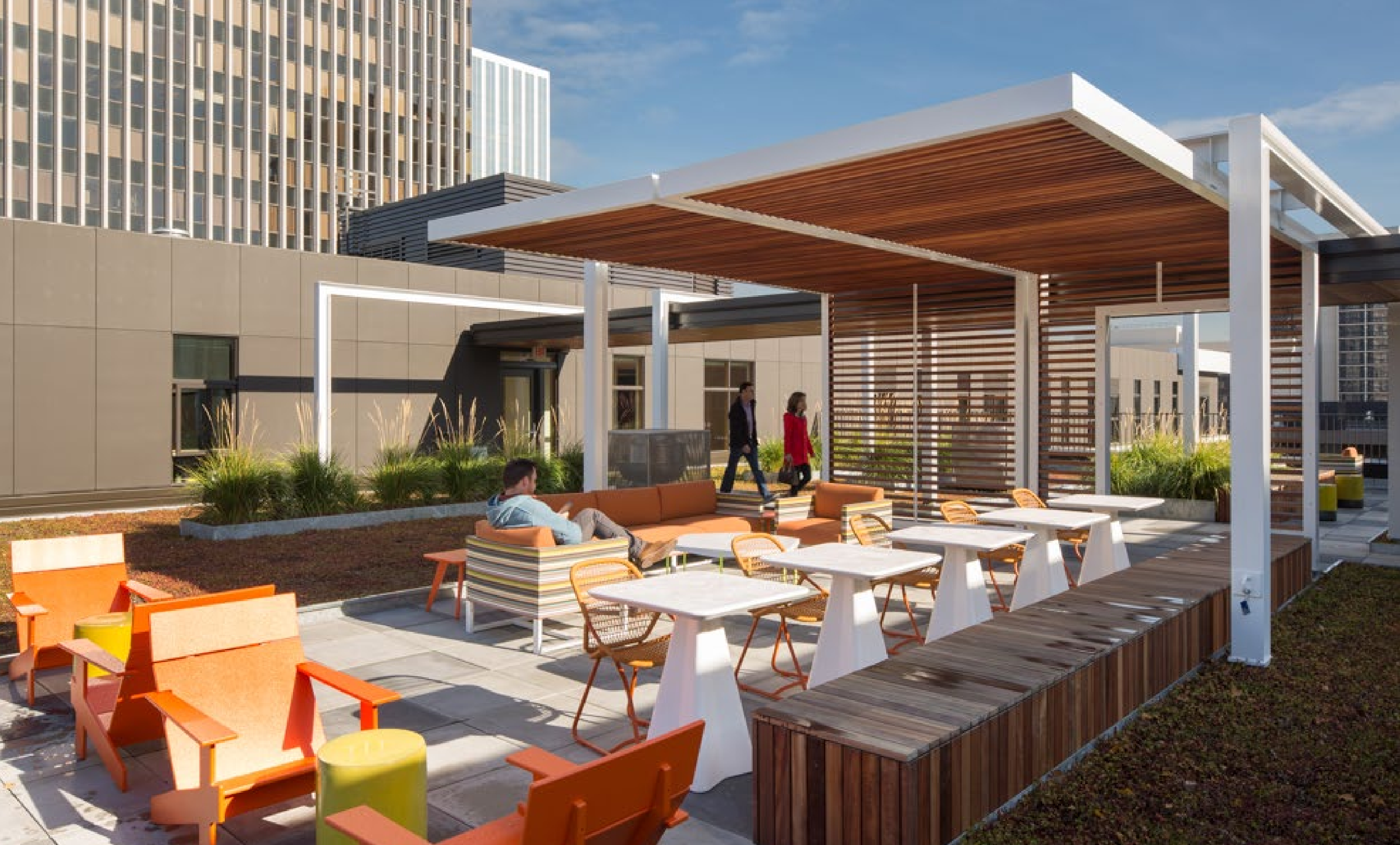
Verdant Eco-Roofs. Eco roofs were used throughout to mitigate heat island effect, insulating the buildings beneath to help reduce energy consumption, while providing a reminder of the larger context and surroundings of the Pacific Northwest.
