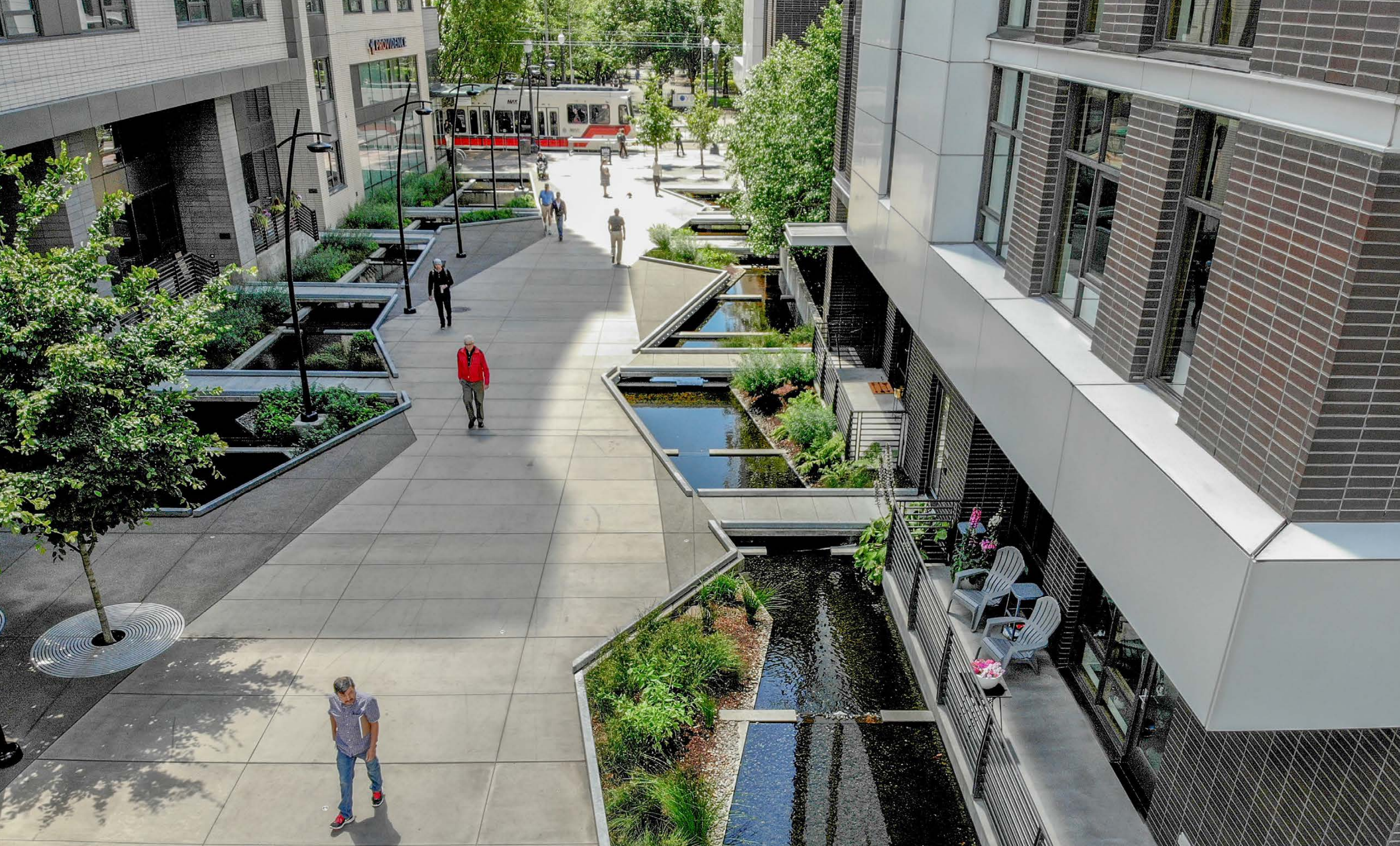
Water Street. The central corridor, collects, conveys, and treats stormwater as part of larger integrated system. Its flowing waterways are sourced from harvested rainwater; its formation brings joy to people and quenches the thirst of the growing urban ecosystem.
