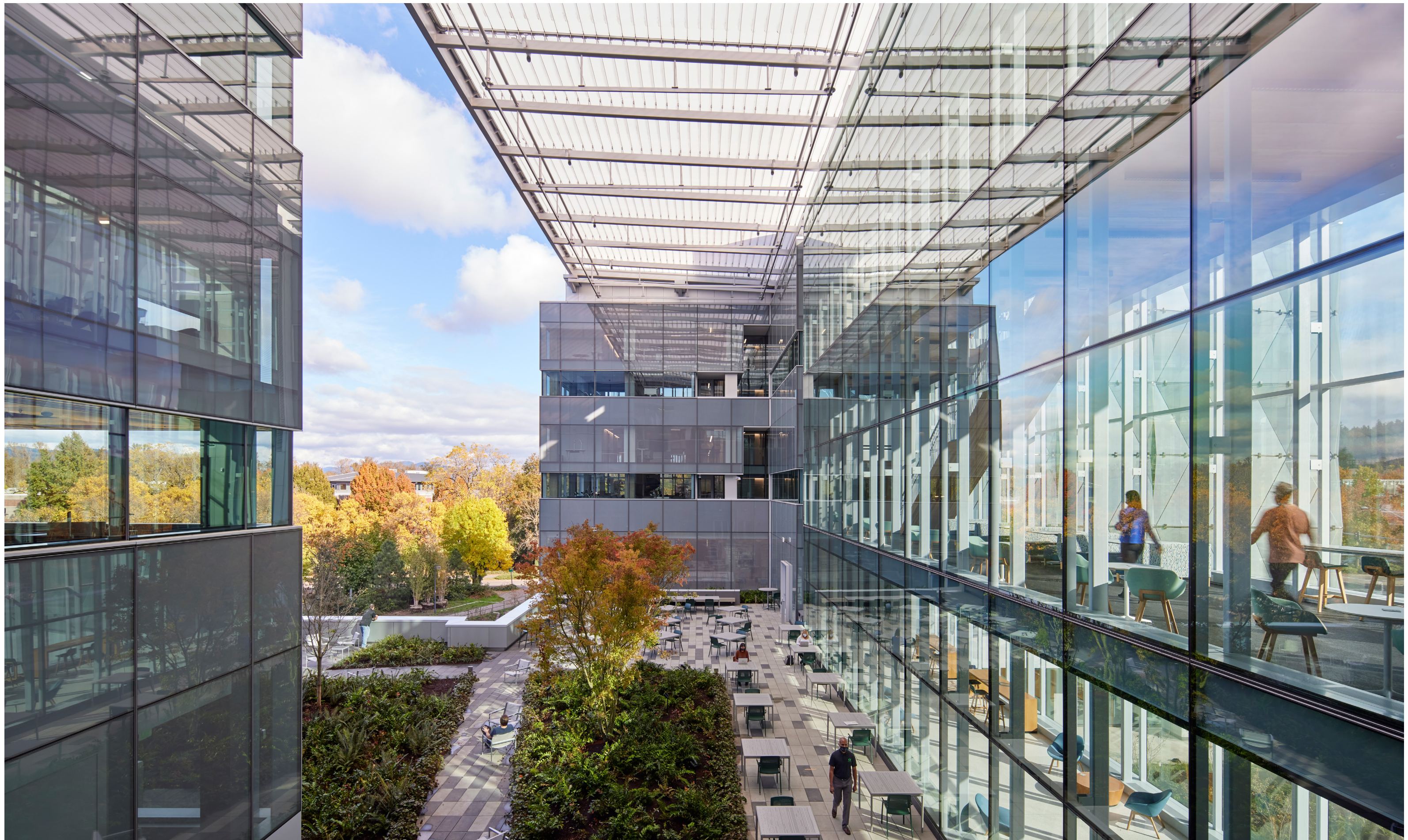
TRANSPARENCY. The University of Oregon's Phil and Penny Knight Campus for Accelerating Scientific Impact encourages innovation through teamwork and transparency. Photo Credit: Bruce Damonte
