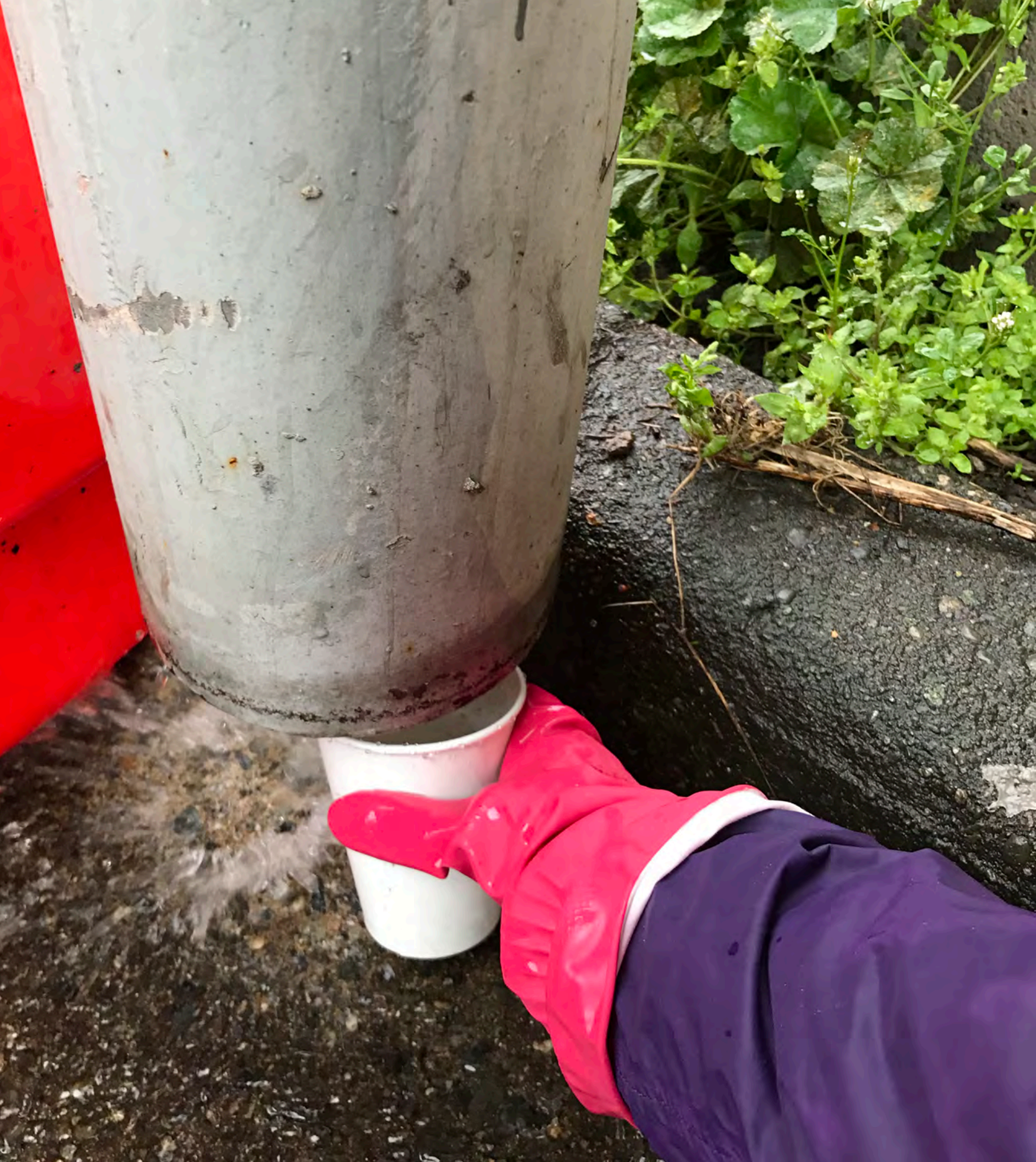
The Aurora Bridge, a state highway, sits over Troll Avenue. Originally, downspouts with toxic runoff from the Bridge were led directly onto the street and down into Lake Union, a major spawning route for the region's Salmon.
