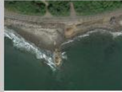
5 WSDOT Dynamic Revetment
