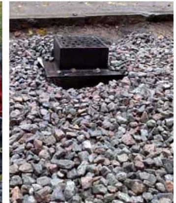
Creation of structural soil for trees in paved area. The pictures show structural skeleton with aerated bearing layer, an air inlet of type TLV 2333 Clarova with cover, addition of planting soil type D and aerated bearing layer around the air vent. (Photo: Orjan Stål).
