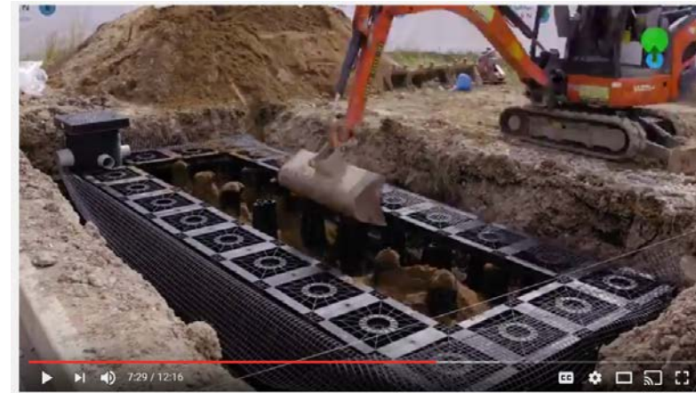
Installing a SUDS Stormwater Urban Drainage System Tree Pit
