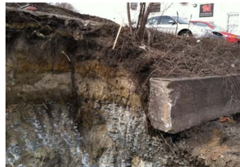
Rooting soil under parking lot
