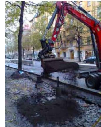
Creation of structural soil for trees in paved area. The pictures show structural skeleton with aerated bearing layer, an air inlet of type TLV 2333 Clarova with cover, addition of planting soil type D and aerated bearing layer around the air vent. (Photo: Orjan Stål).
