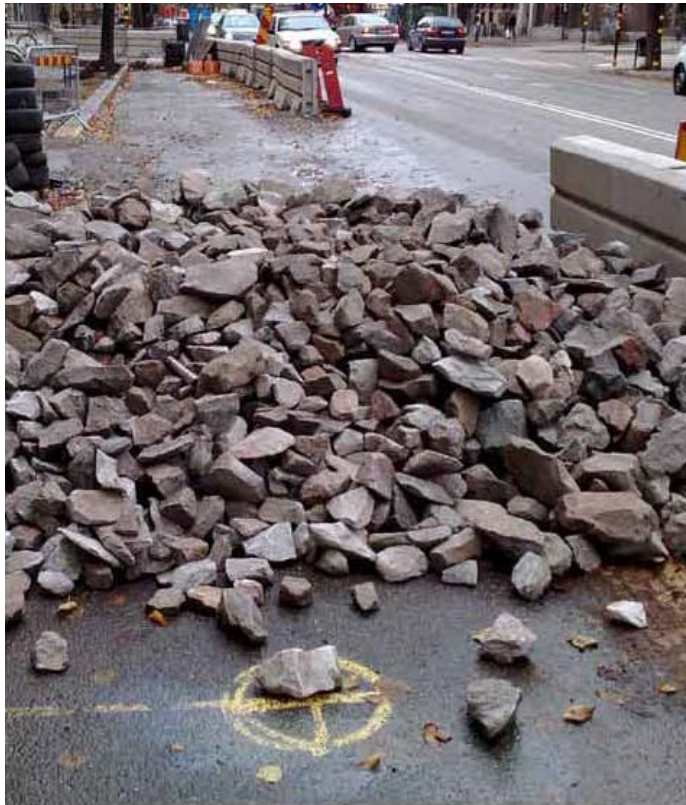
Structural material, 100-150mm crushed rock for structural soil. (Photo: Örjan Stål)
