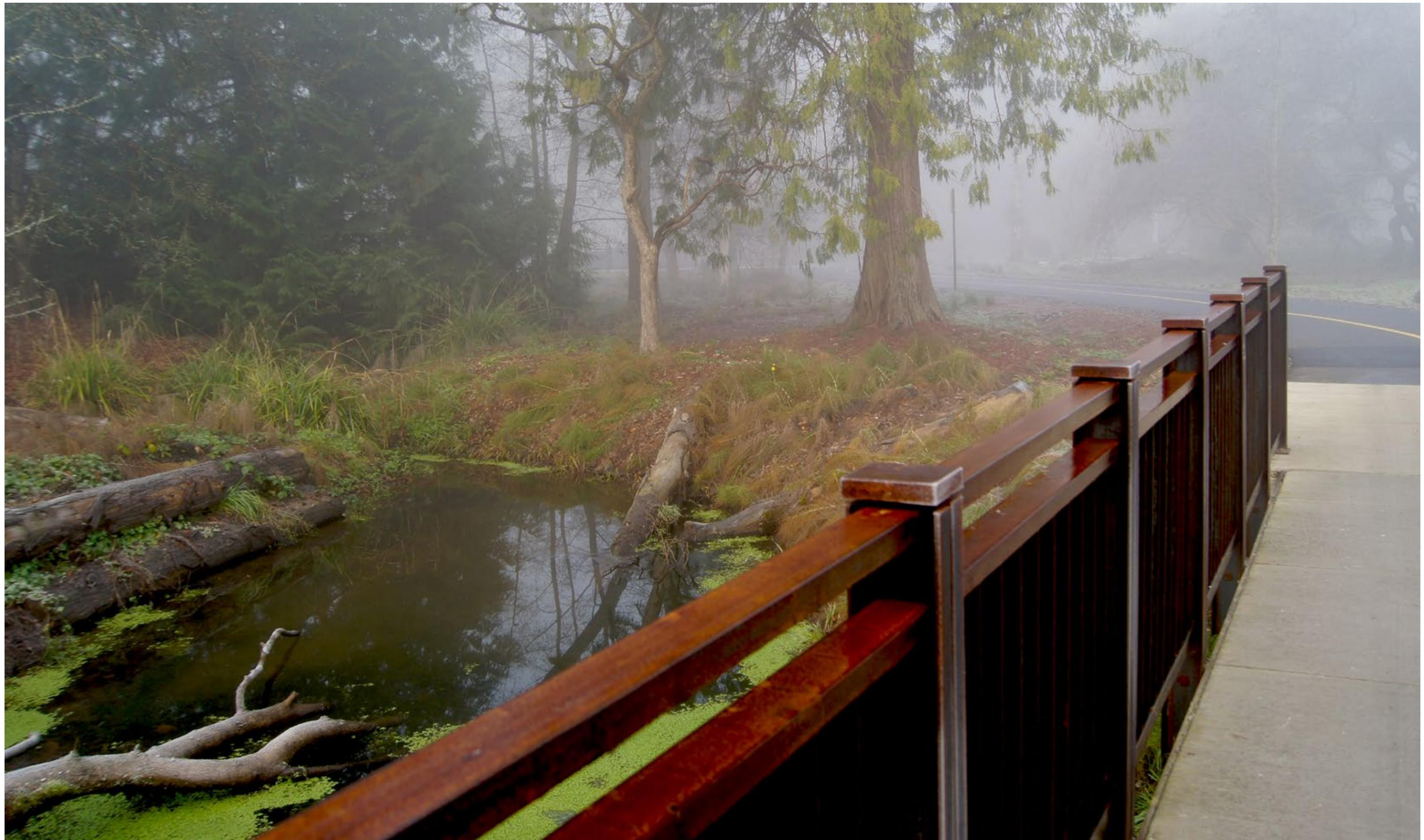
Although not certified under a rating system, sustainability drove materials selections. Using weathering steel for bridges and railings instead of standard galvanized or painted steel prevented zinc and paint from entering the stream. Irrigation piping was HDPE instead of PVC.
