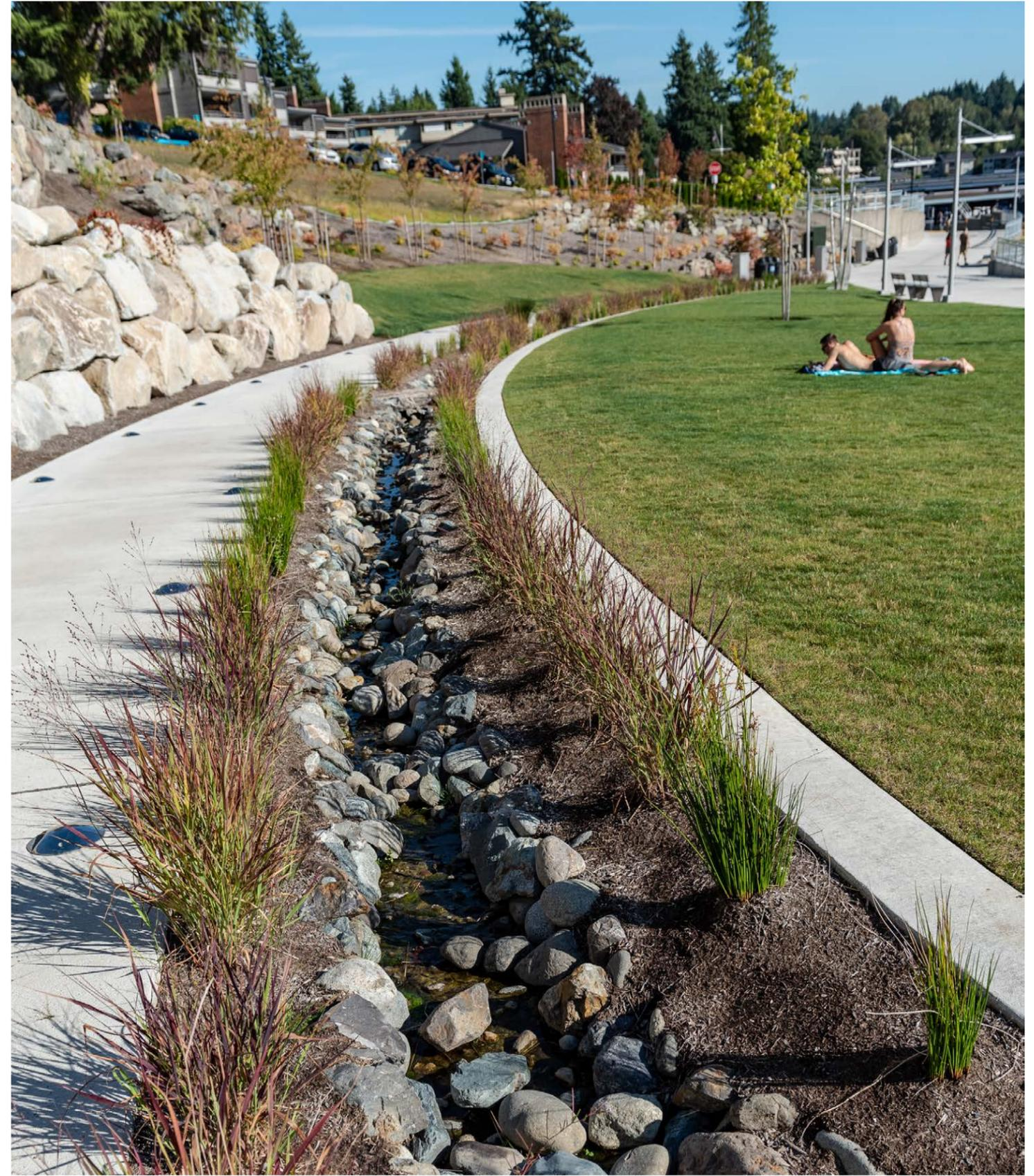
A 300-foot-long restored stream channel (left) replaces a buried stormwater pipe, improving water quality and habitat. An open, cobble-lined channel (right) infiltrates and conveys treated stormwater from the new parking area to the lake.
