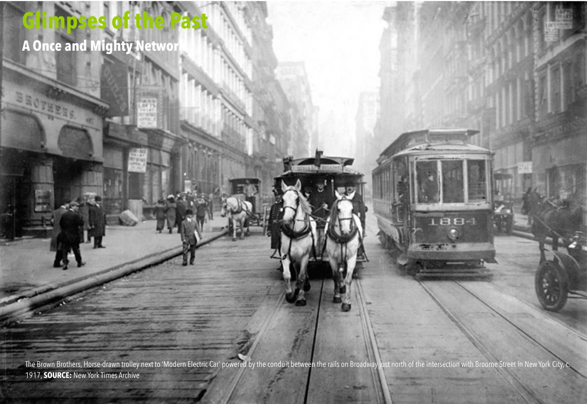
The Brown Brothers, Horse-drawn trolley next to 'Modern Electric Car' powered by the conduit between the rails on Broadway just north of the intersection with Broome Street in New York City, c. 1917, **SOURCE:** New York Times Archive
