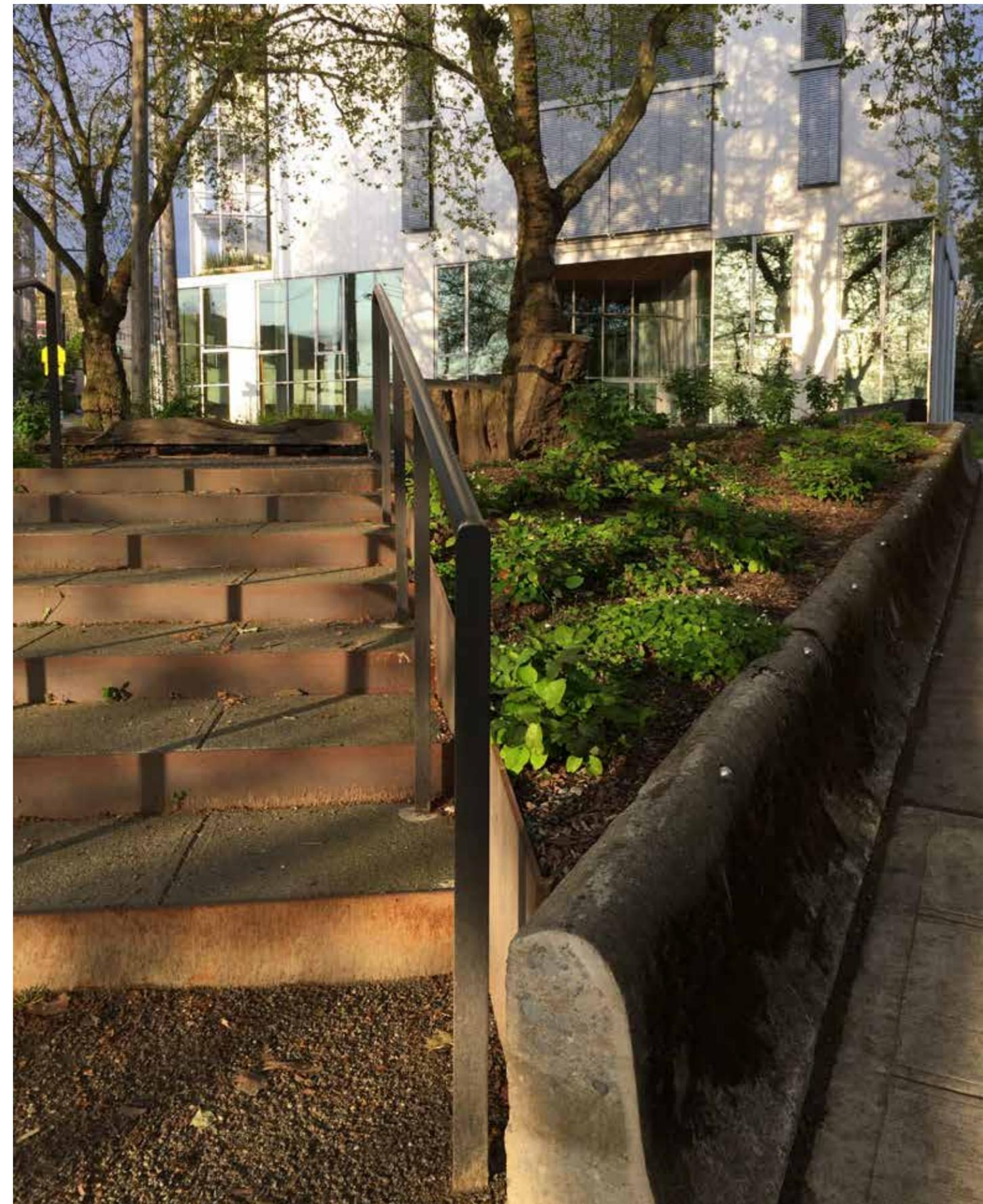
The design preserved the existing raised concrete planter walls but strategically removed two sections enabling barrier-free access into center of the tree canopy. Removed sections were retained onsite as remnants and reinforce the concept of material salvage and reuse.
