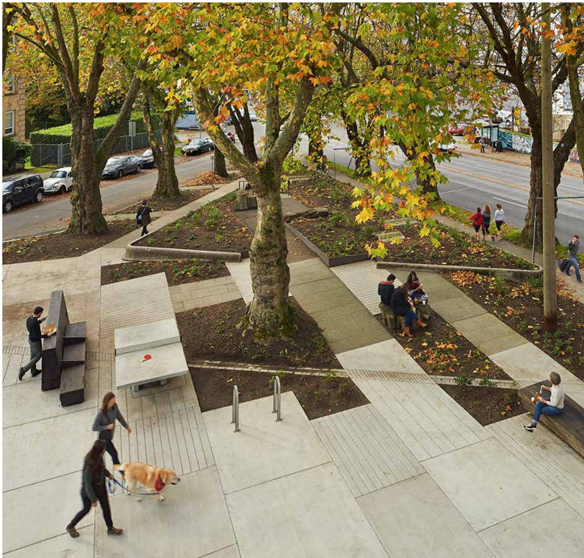
Curbless space is open to only non-motorized uses aside from emergency vehicles. New hardscape and grading required surgical insertion between existing trees. Every piece of existing hardscape in park was salvaged and reused onsite.
