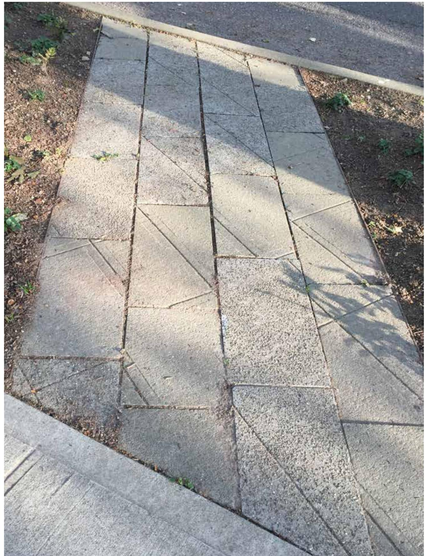
Existing concrete sidewalks crowding the trees were salvaged for reuse. The concrete was sawcut into new large- and small-scale modules and reinstalled onsite to serve as pavers and stair treads.
