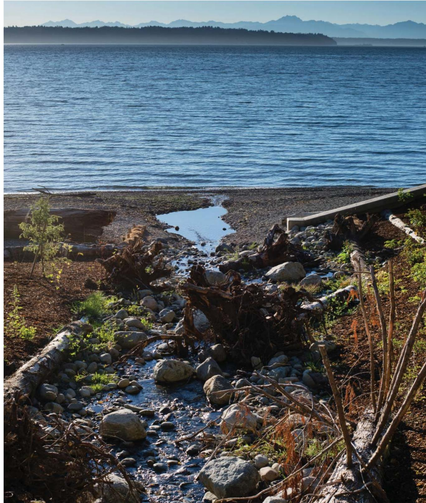
The restored, daylighted stream near the Environmental Science Center building provides 30 cubic yards of natural beach-material delivery each year. This material, formerly a maintenance problem that was trucked off site, now adds to the long-term sustainability of the project.
