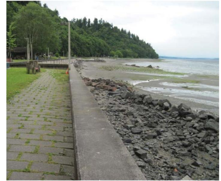
Armoring increases wave reflectivity and erosion, leading to more armor.
