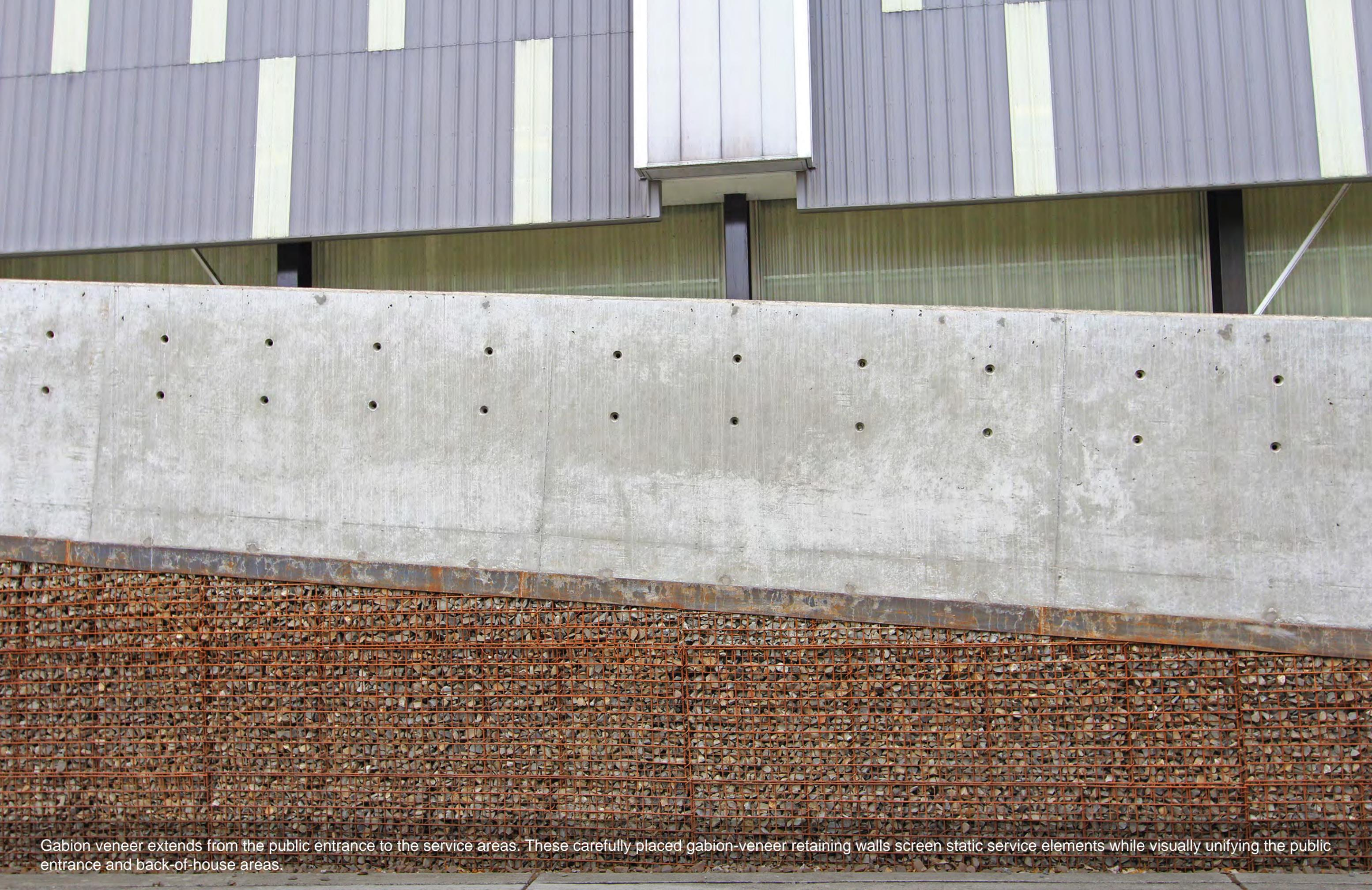
Gabion veneer extends from the public entrance to the service areas. These carefully placed gabion-veneer retaining walls screen static service elements while visually unifying the public entrance and back-of-house areas.
