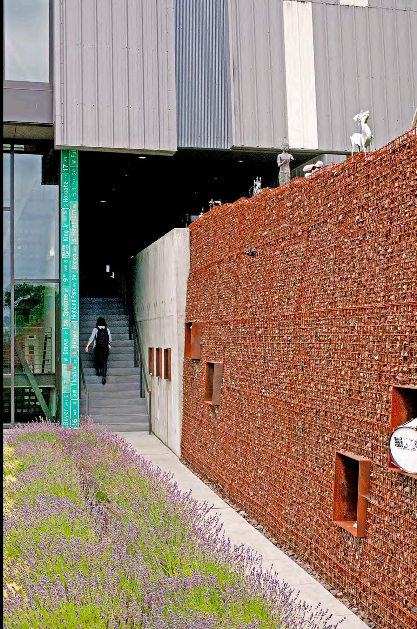
The site design includes over 600 linear feet of custom gabion veneer walls. Their highly textured presence are designed at a scale to draw interest from vehicles on adjacent roadways and from pedestrians on the site.
